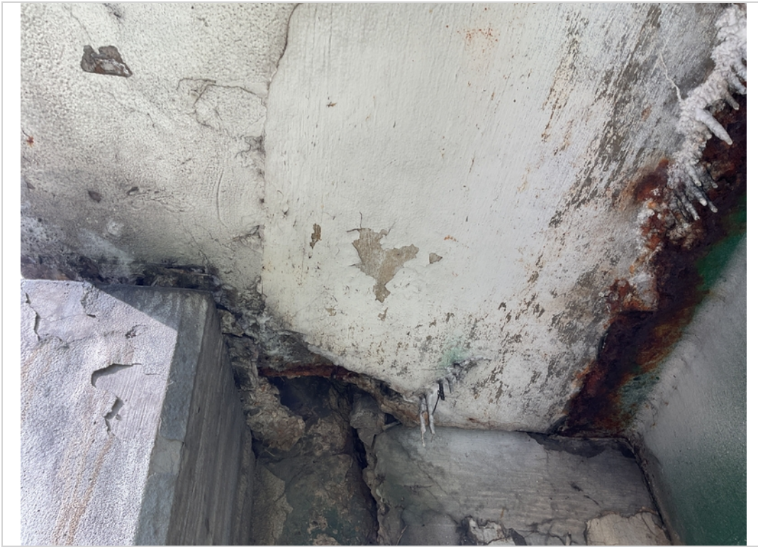
Overhang span 1 right side spall with exp steel
