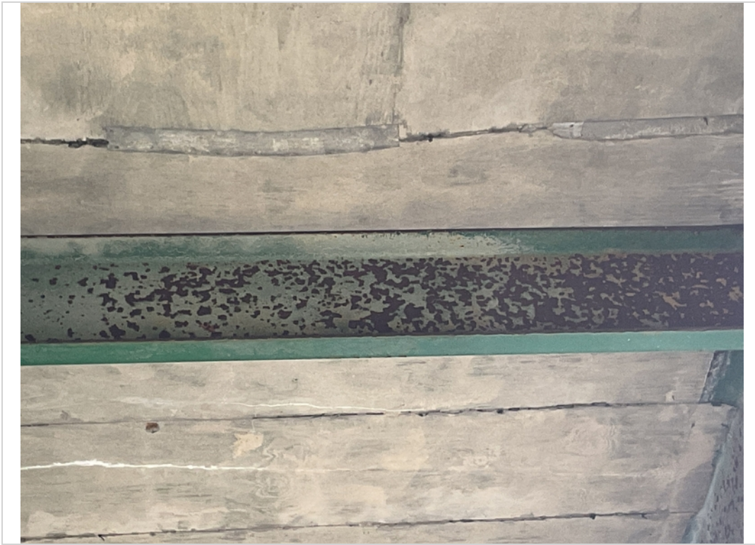
Span 2 diaphragm #2 corrosion
