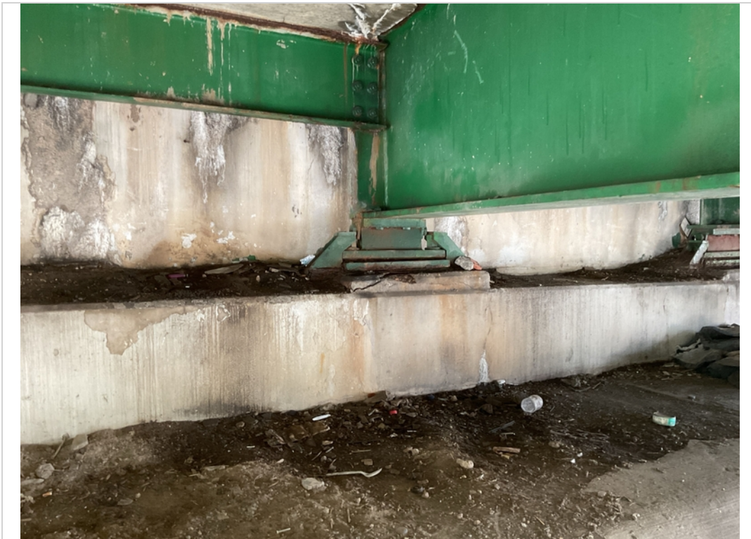
Abut 1 bearing C cracked riser and corrosion
