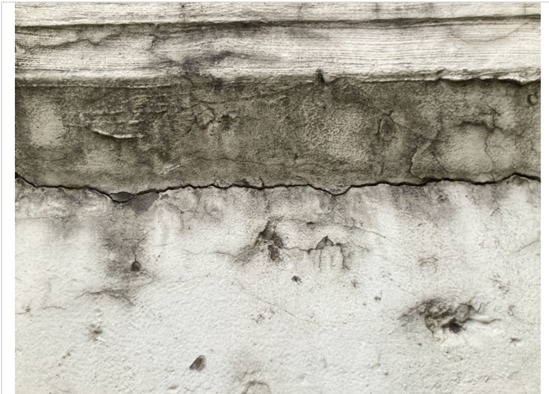
Parapet left cracks
