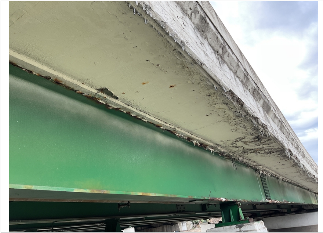
Overhang span 3 left side scale with eff
