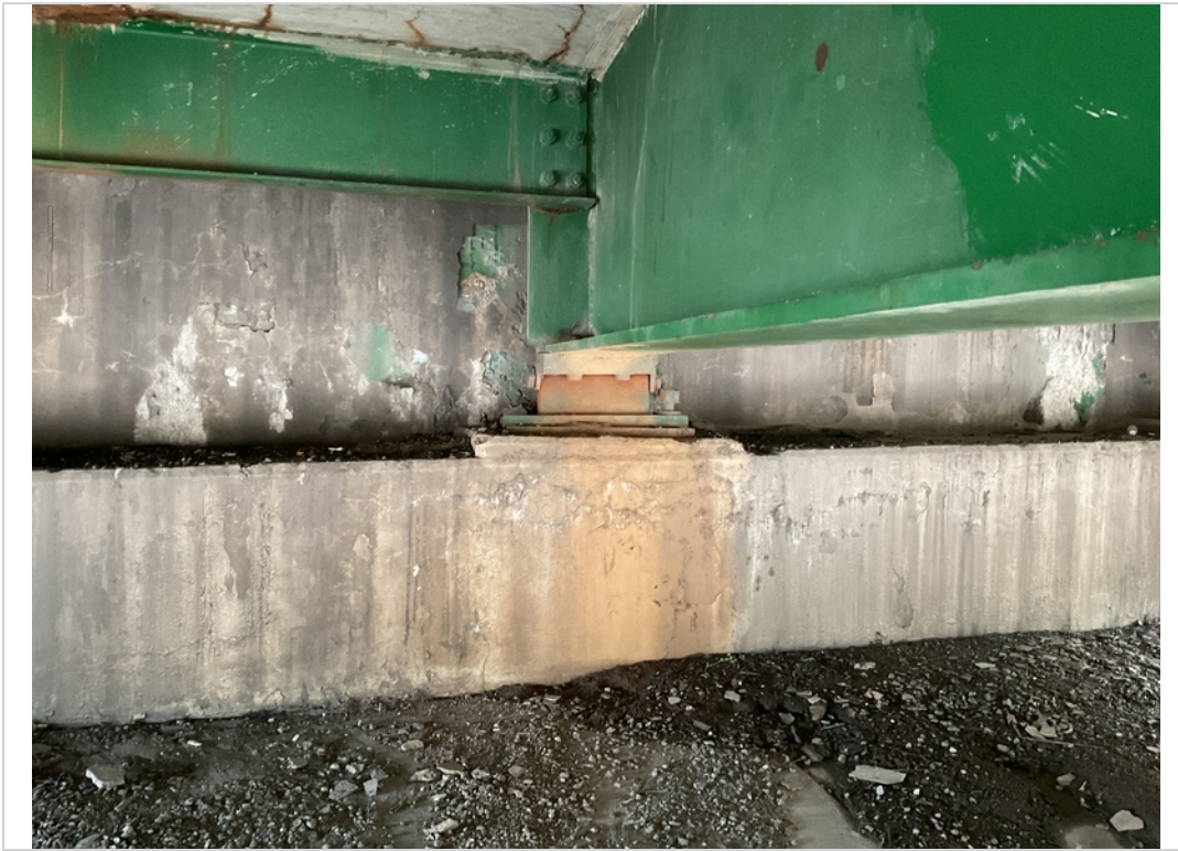
Abut 2 Bearing C missing bolt loose anchorage corrosion
