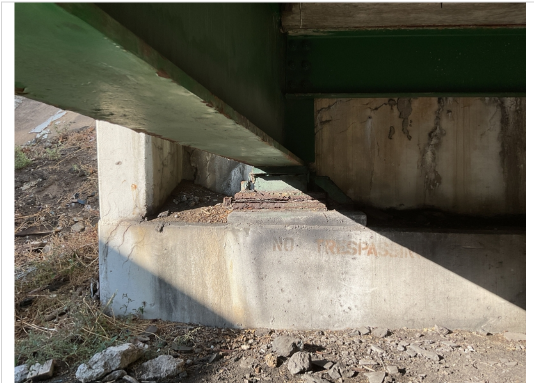
Abut 1 bearing E missing stabilizer arm
