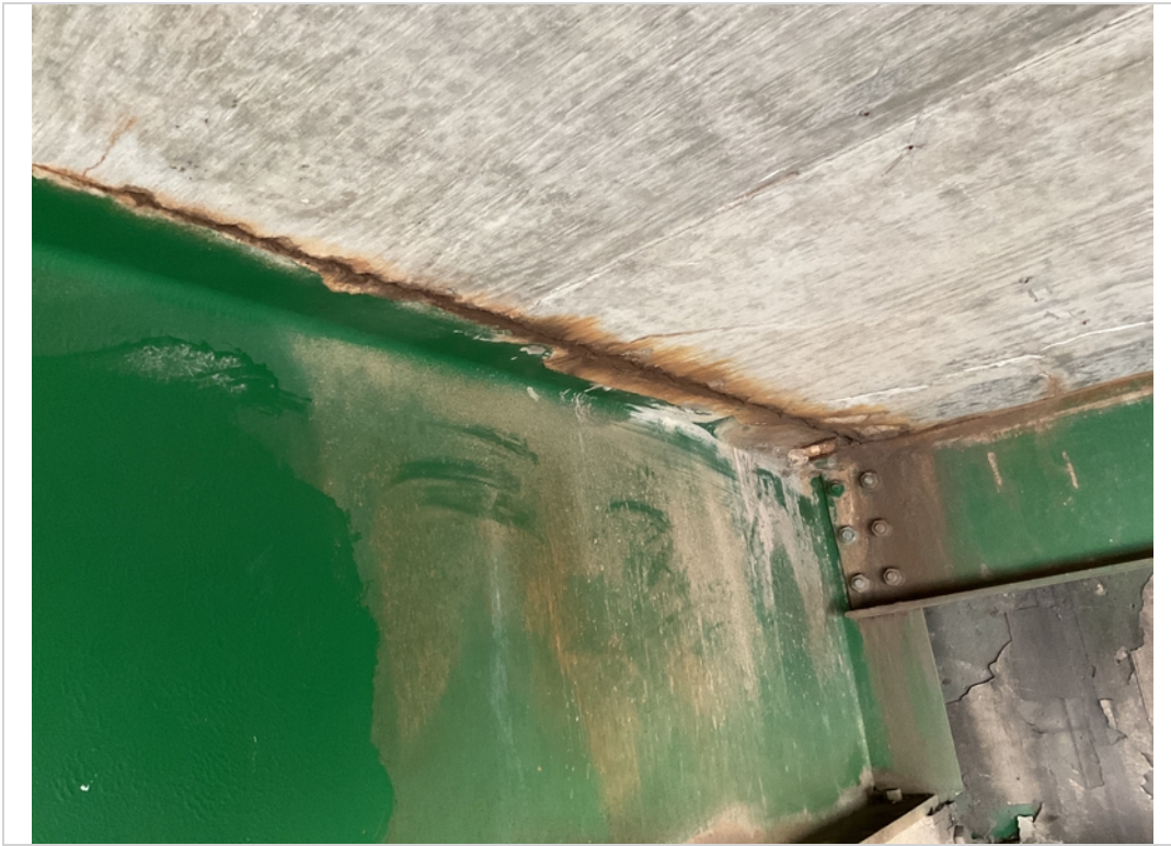
Span 3 Girder B top flange corrosion
