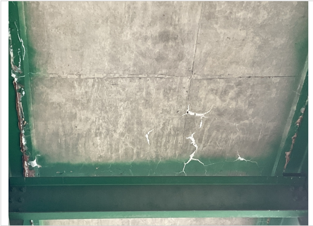
Span 2 bay C random map cracks with eff
