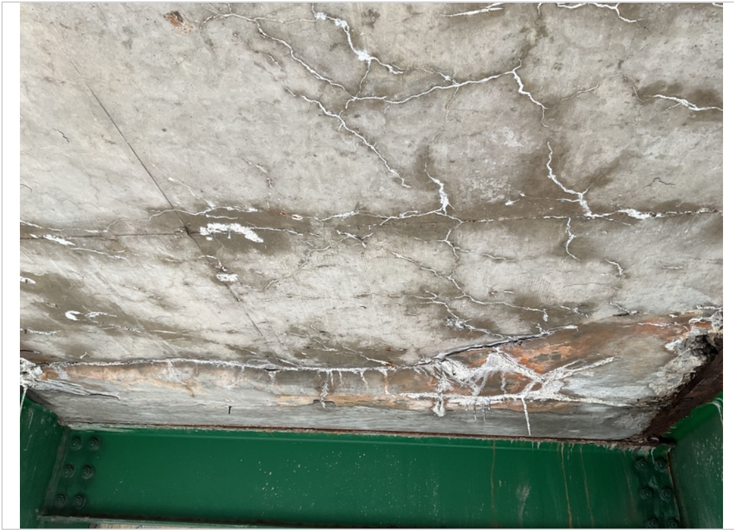
Span 1 bay D failing patch with eff
