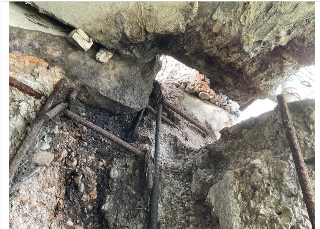
Overhang at Abut 1 left side and spall w/exp steel
