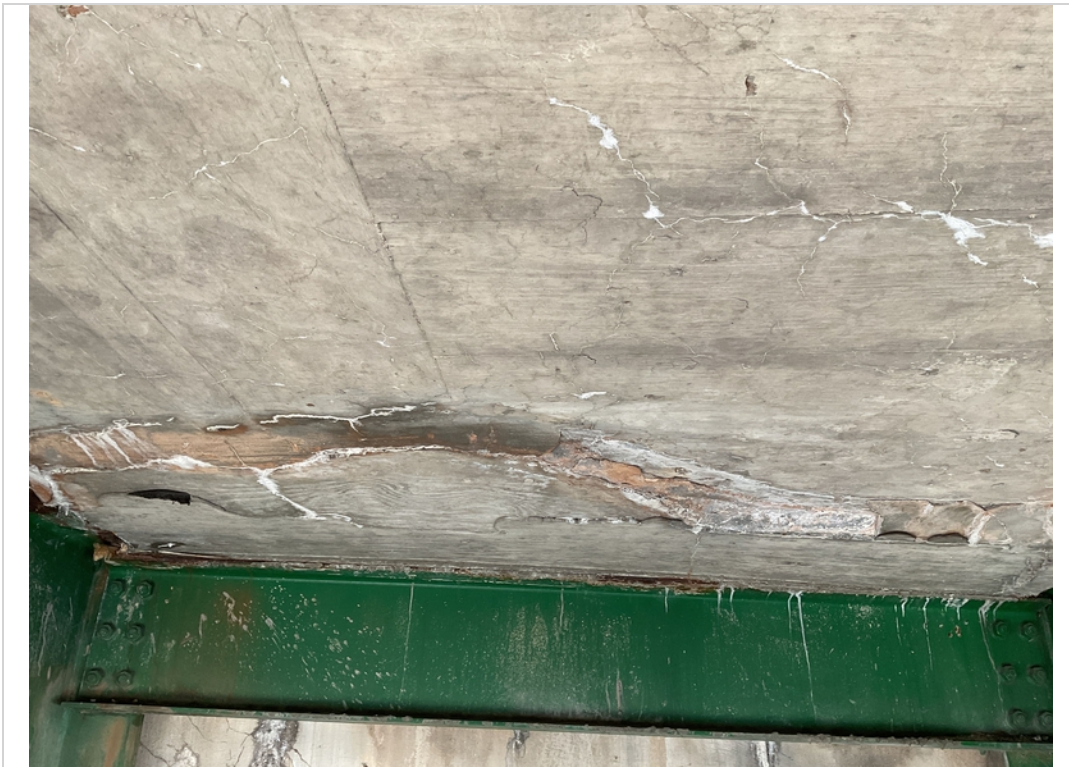
Span 1 bay B failing patch with eff
