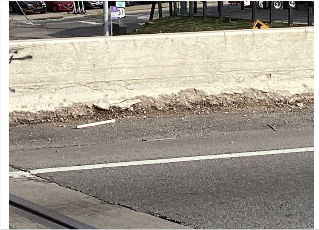
Span 1 and 2 parapet left heavy scale
