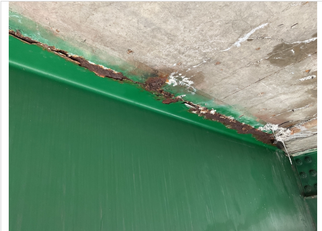
Span 1 Girder E top flange corrosion
