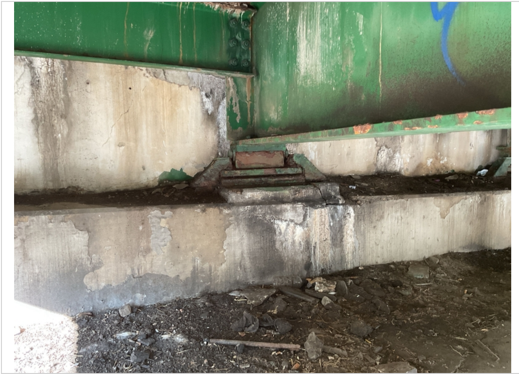
Abut 1 bearing D corrosion and cracked riser. W/eff
