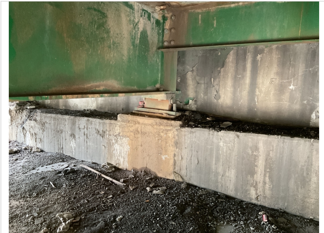
Abut 2 bearing B loose anchorage. Missing nut corrosion
