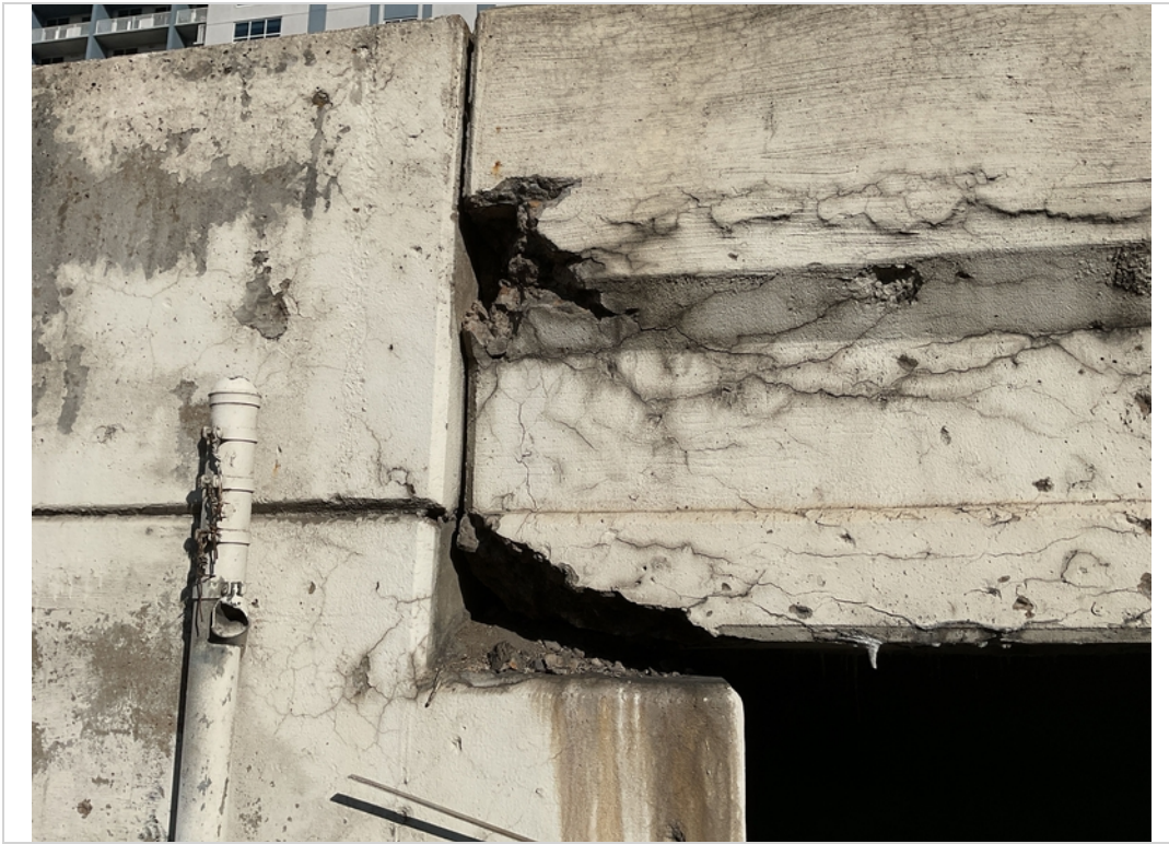
Bridge rail span 1 spall
