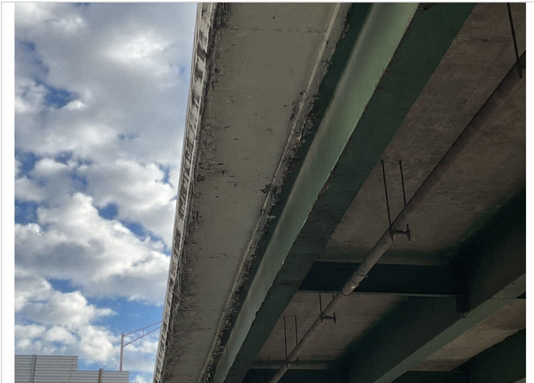
Overhang span 2 left side map cracks with eff
