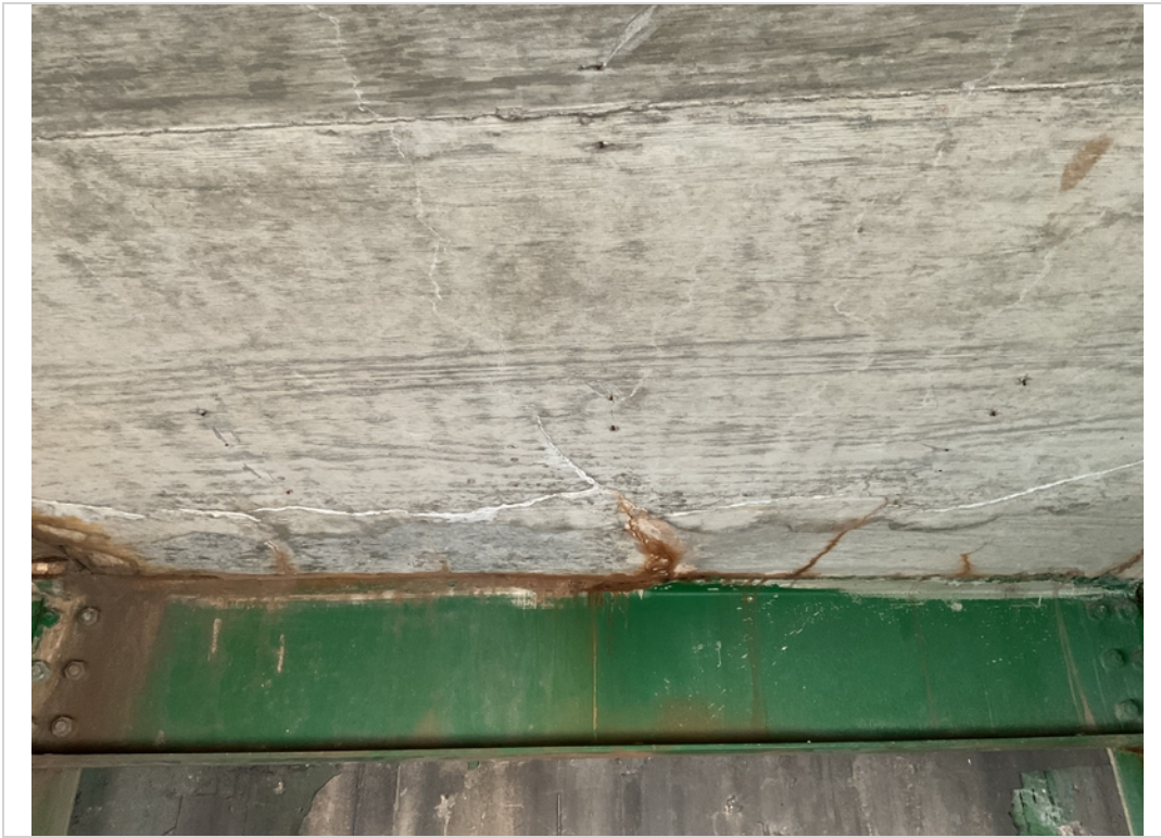
Span 3 bay B failing patch with eff
