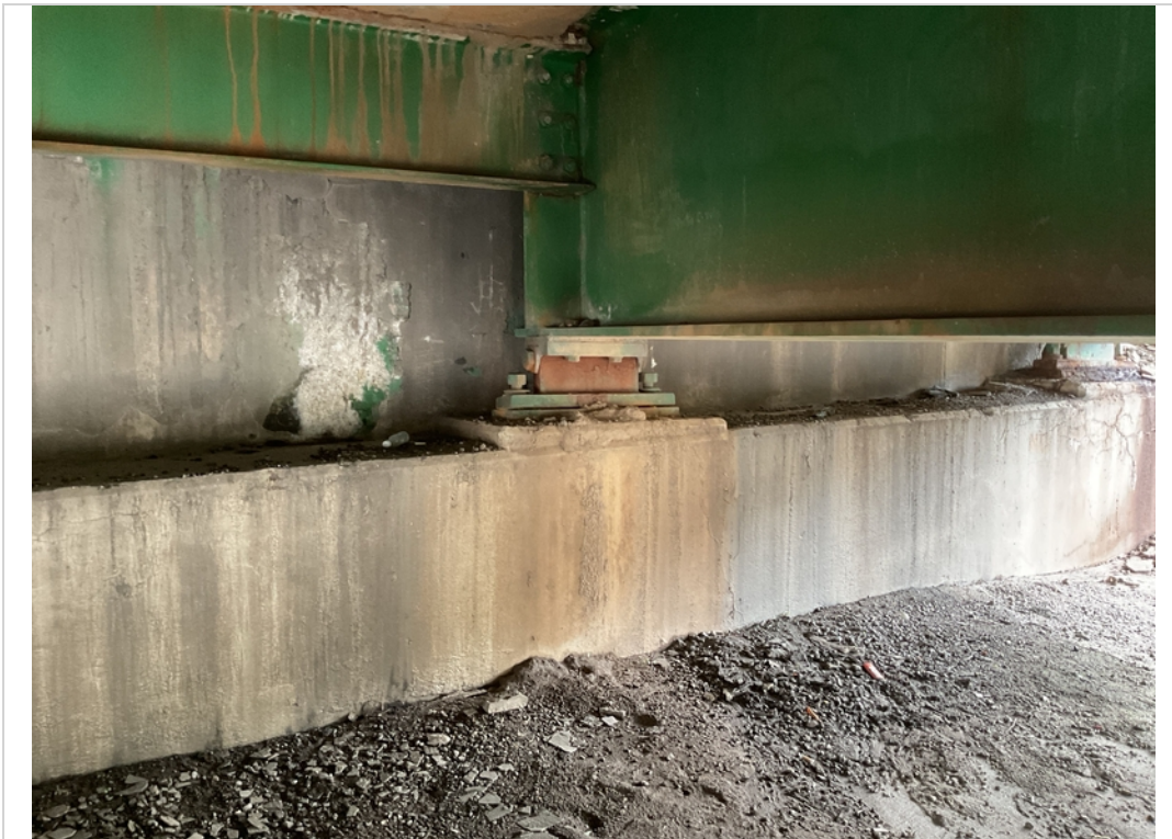
Abut 2 Bearing B corrosion loose anchorage
