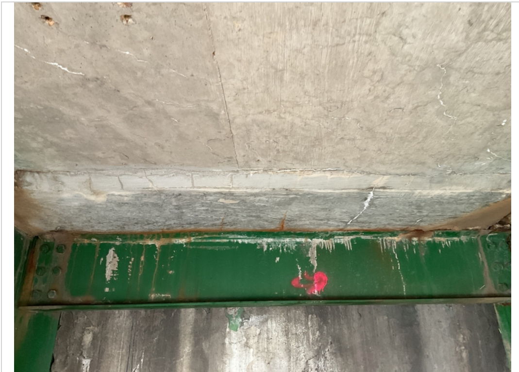
Span 3 bay A failing patch will eff
