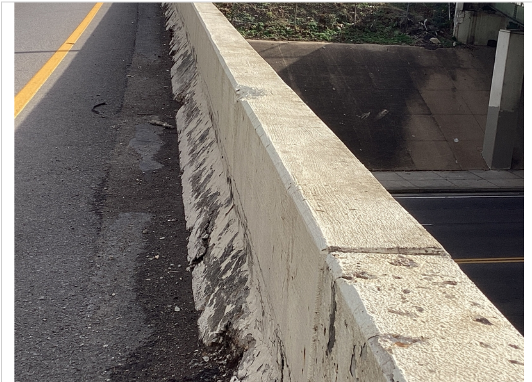
Span 1 parapet right spall
