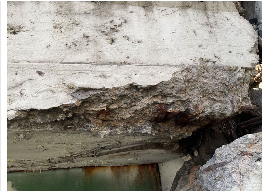
Overhang span 1 heavy scale with exp steel
