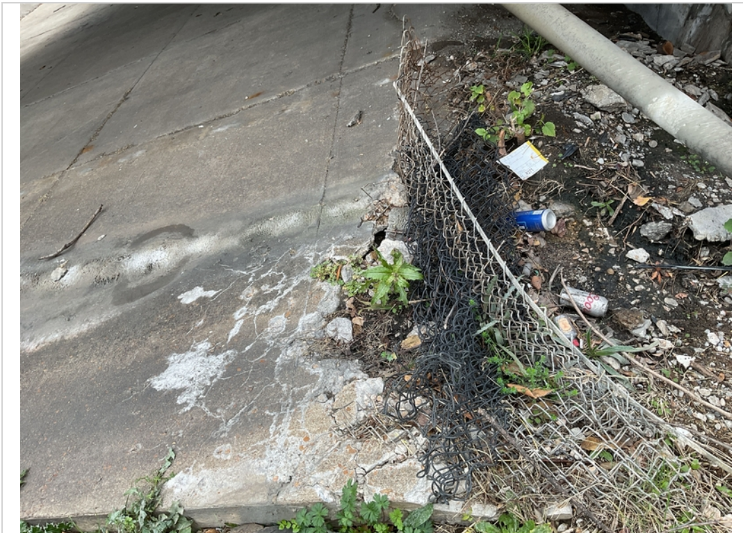
Abut 1 slope cracked w/erosion under slope.
