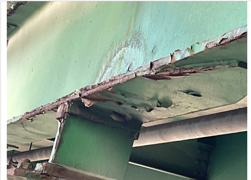
Span 1 Girder A bottom flange corrosion
