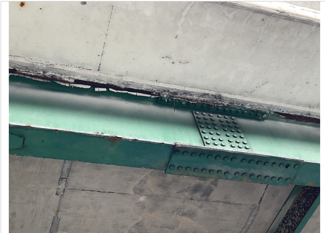
Span 2 Girder E top flange corrosion
