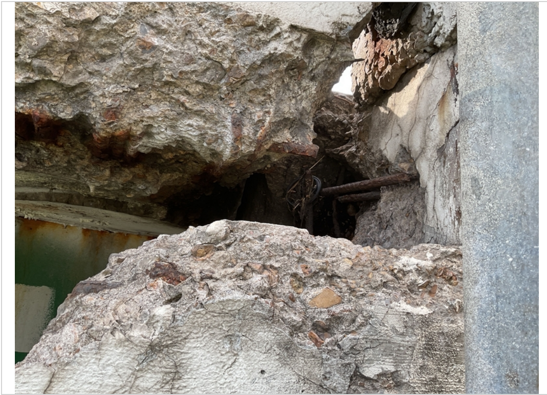
Abut 1 left overhang and back wall spalls w/exp steel and hvy scale
