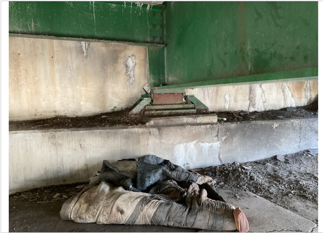
Abut 1 bearing B corrosion vert h.c horiz crack w/eff
