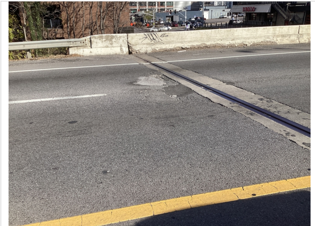
A approach pavement patches depression
