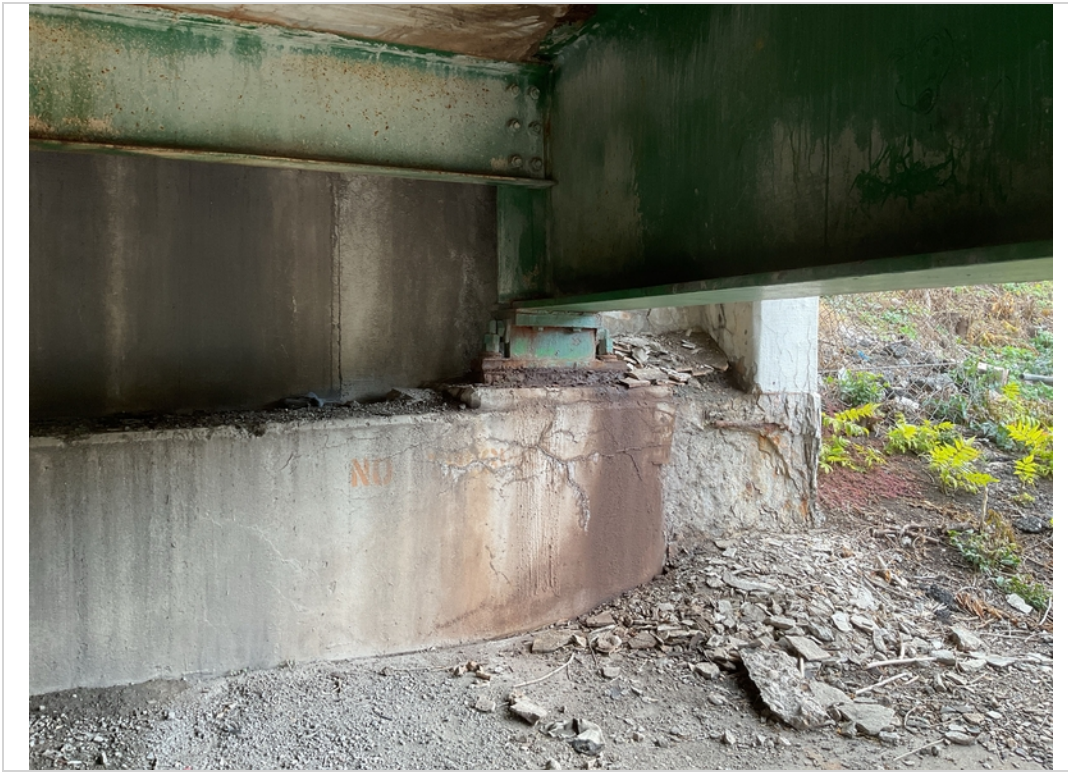
Abut 2 bearing A loose anchorage all bearings rocked rack w/ Hvy debris
