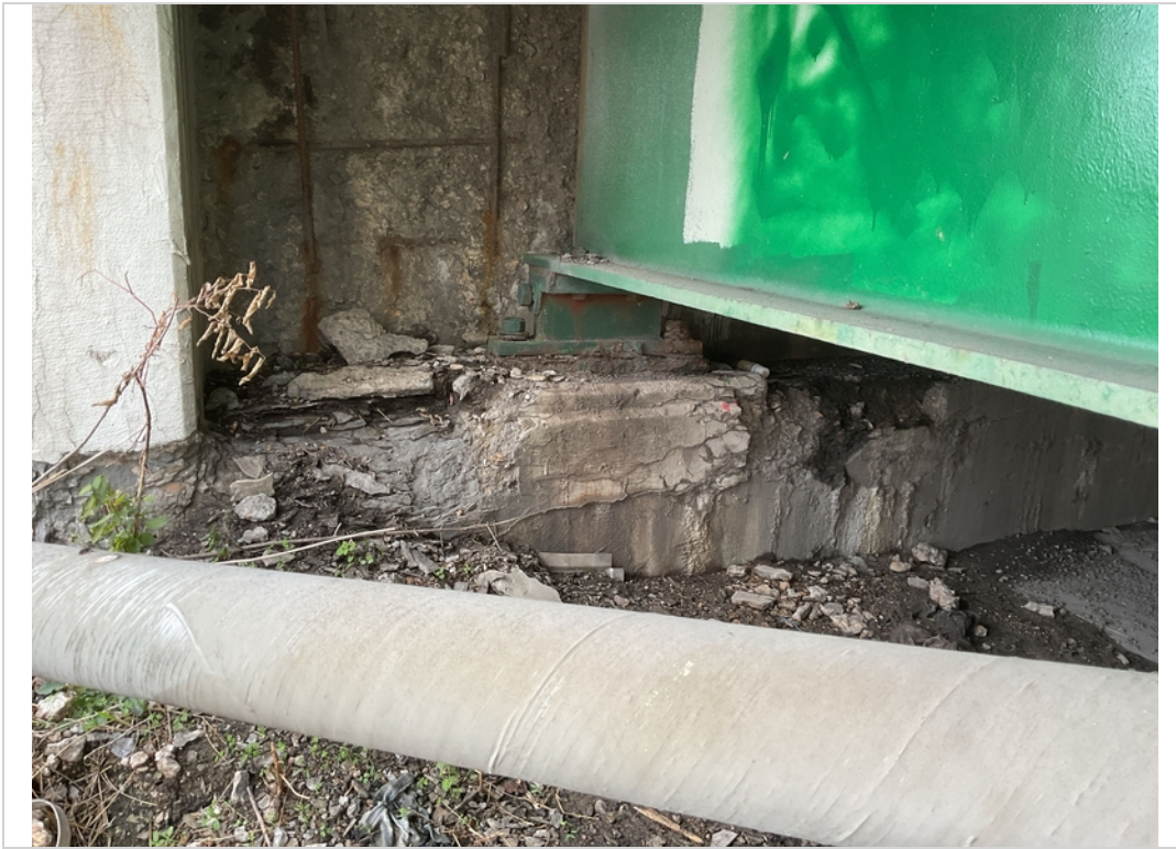
Abut 2 bearing A corrosion.
