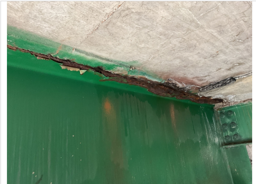
Span 1 Girder D top flange corrosion
