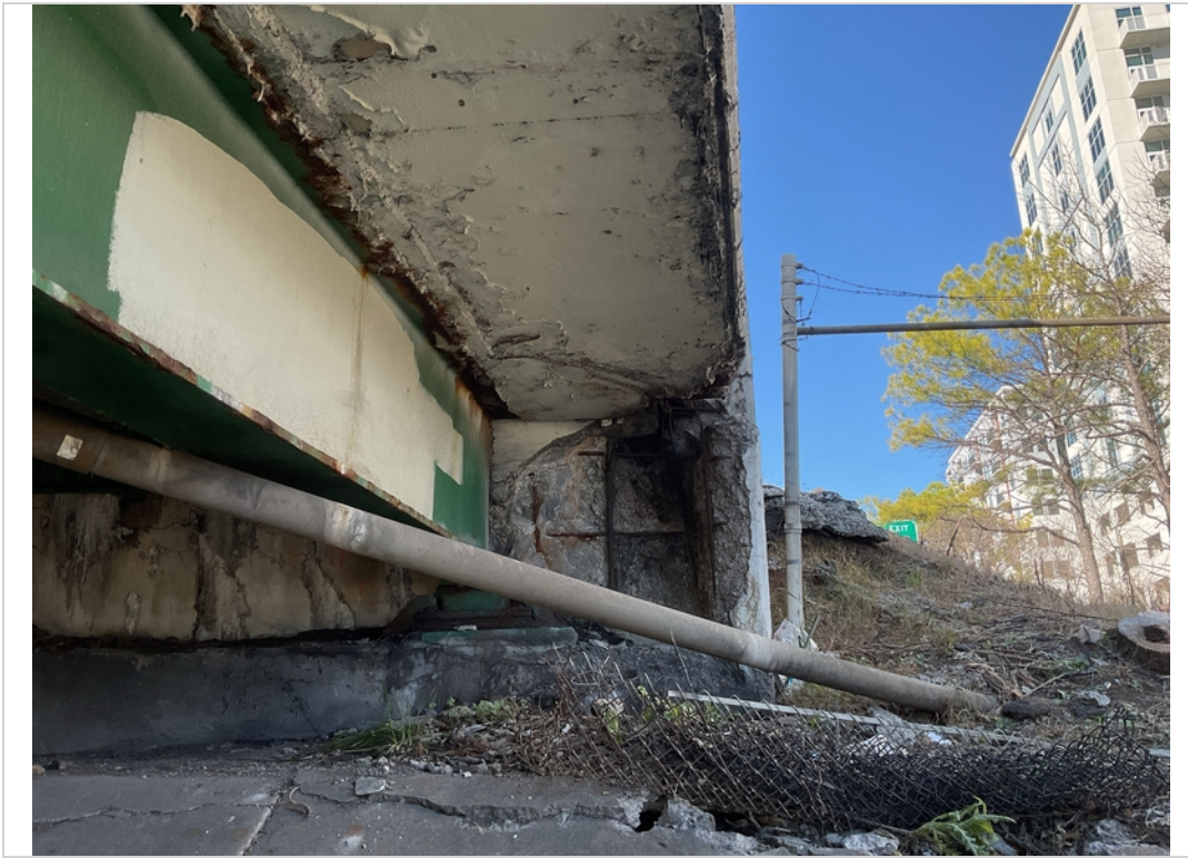
Abut 1 left @left wing hvy scale w/exp steel
