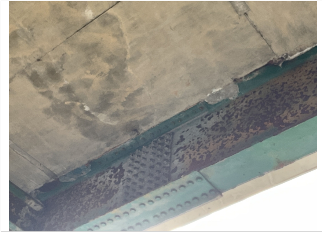
Span 2 Girder E corrosion
