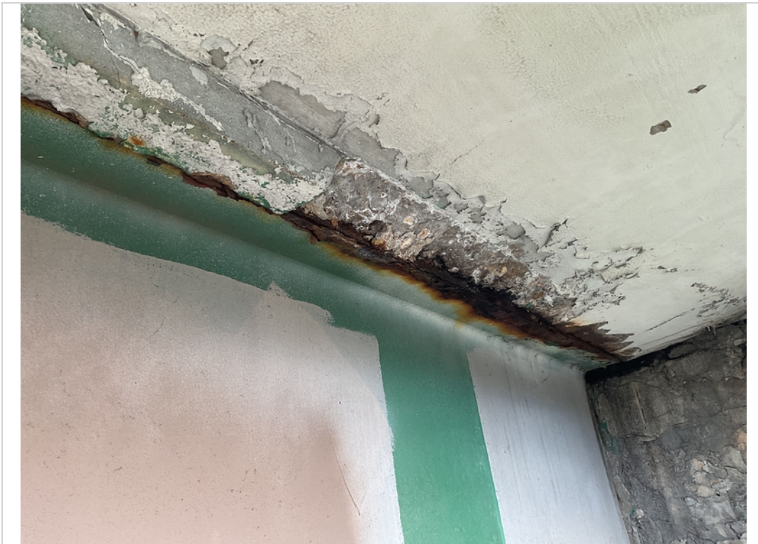
Span 3 Girder E top flange corrosion
