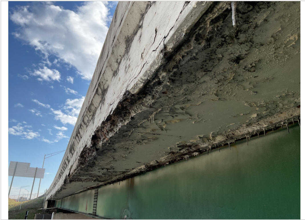
Overhang span 1 left side heavy scale with eff
