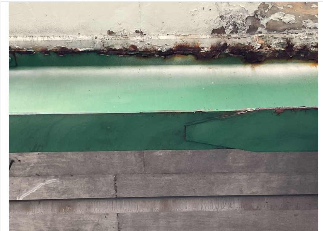
Span 2 Girder A top flange corrosion
