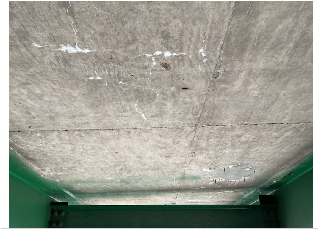
Span 1 bay B random map cracks with eff
