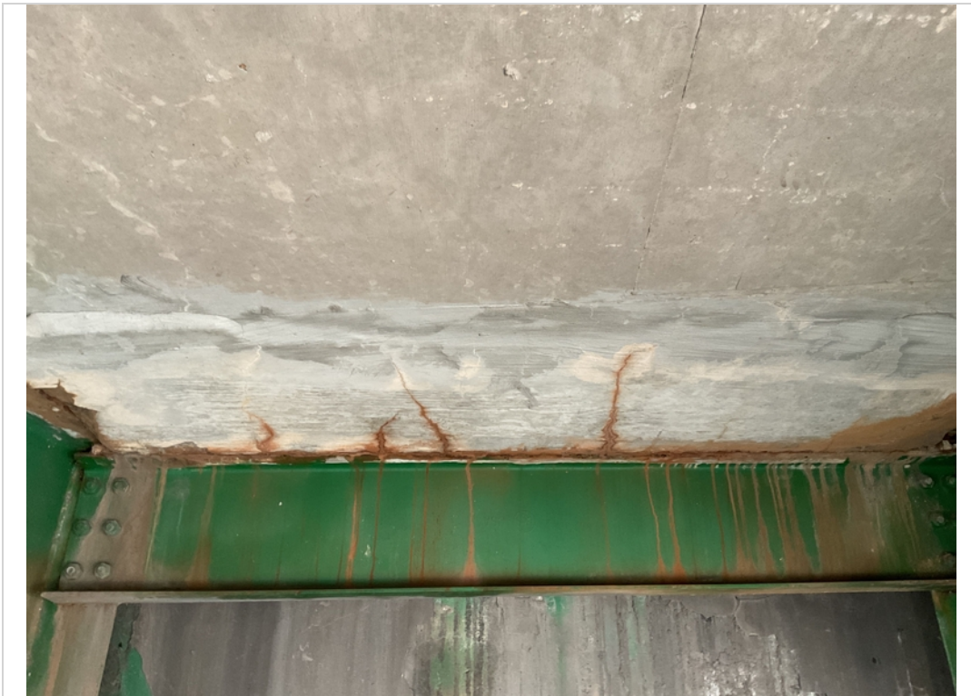
Span 3 bay C failing patch with eff
