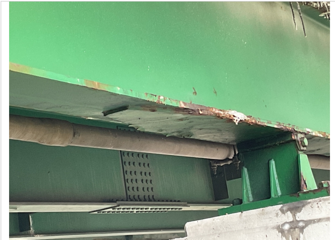
Span 3 Girder A bottom flange corrosion
