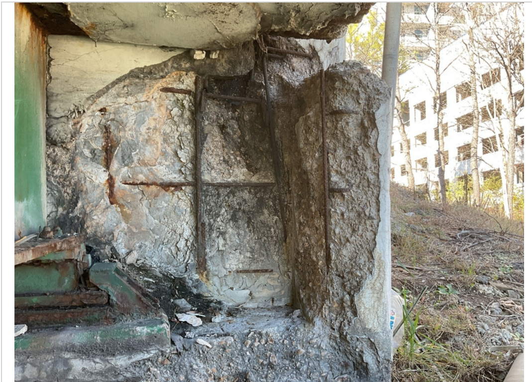
Abut 1 left hvy scale W/exp steel
