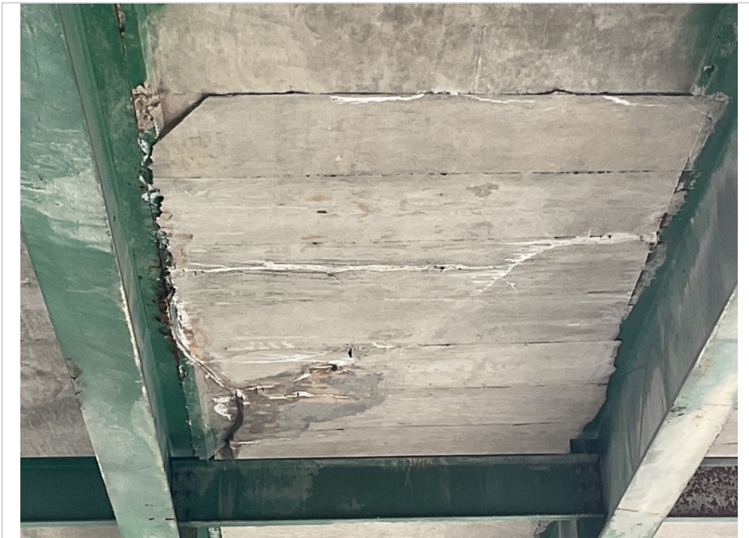
Span 2 bay C failing patch with eff
