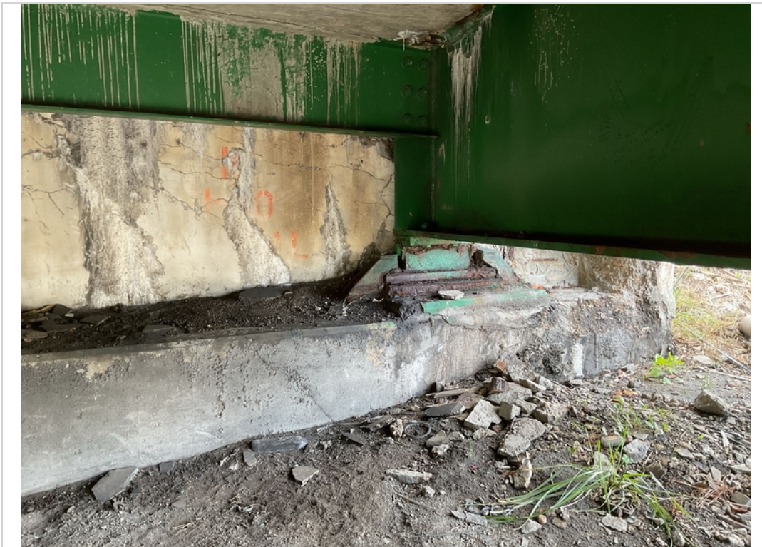
Abut 1 bearing A corrosion all bearing rocked back
