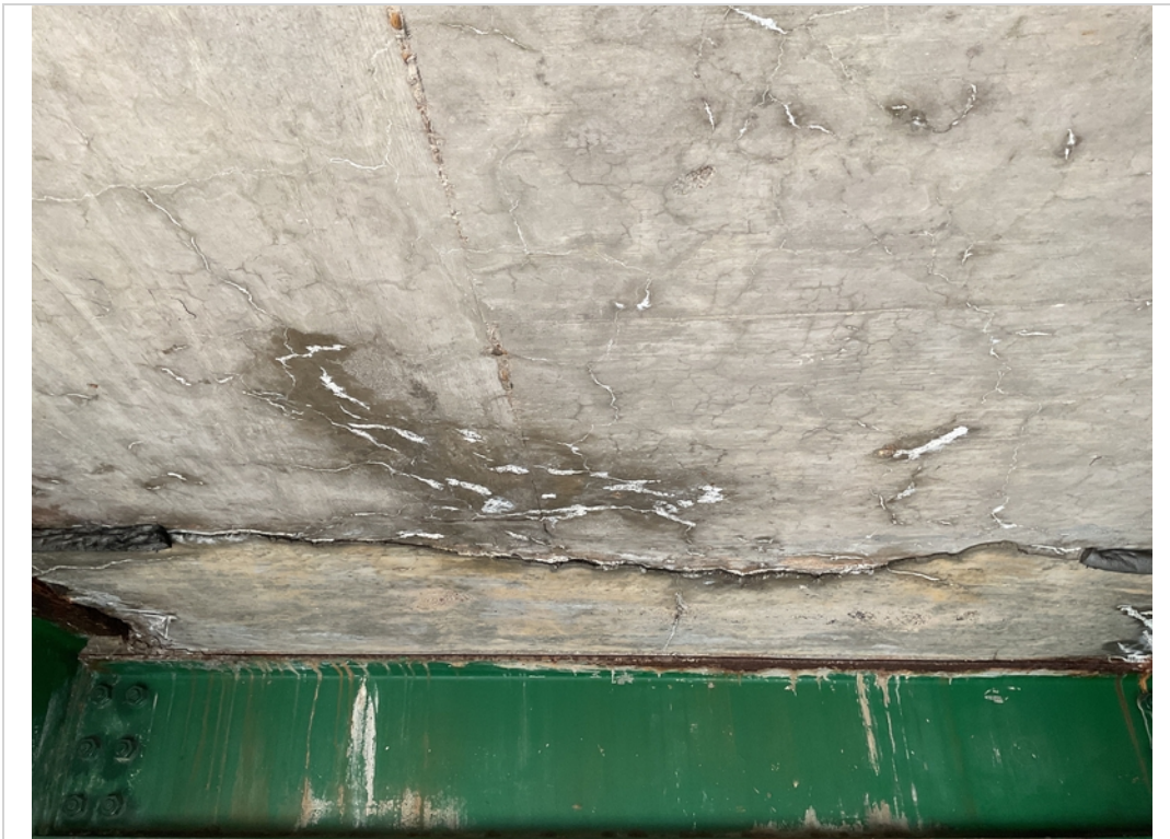
Span 1 bay C random map cracks with eff
