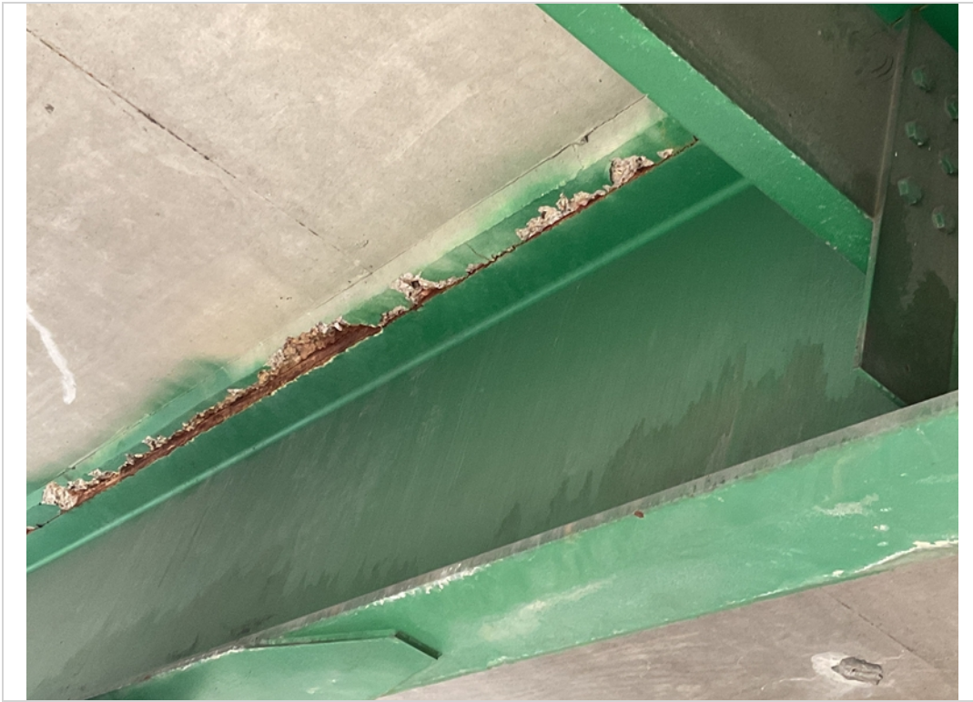
Span 3 bay D spalling at top flange of C
