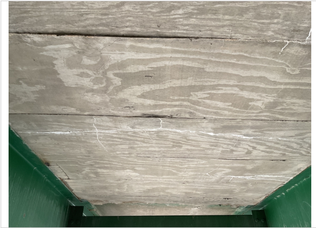
Span 3 bay C random map cracks with eff
