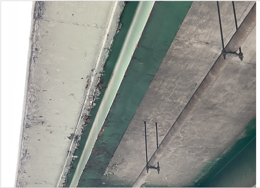
Span 2 Girder A impact scrapes
