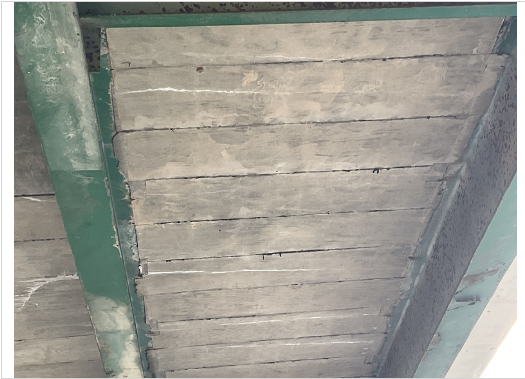
Span 2 bay D random trans cracks with eff
