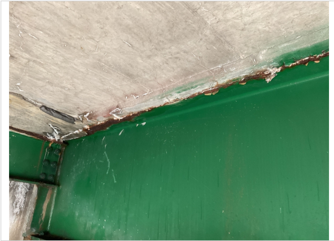
Span 1 Girder C top flange corrosion
