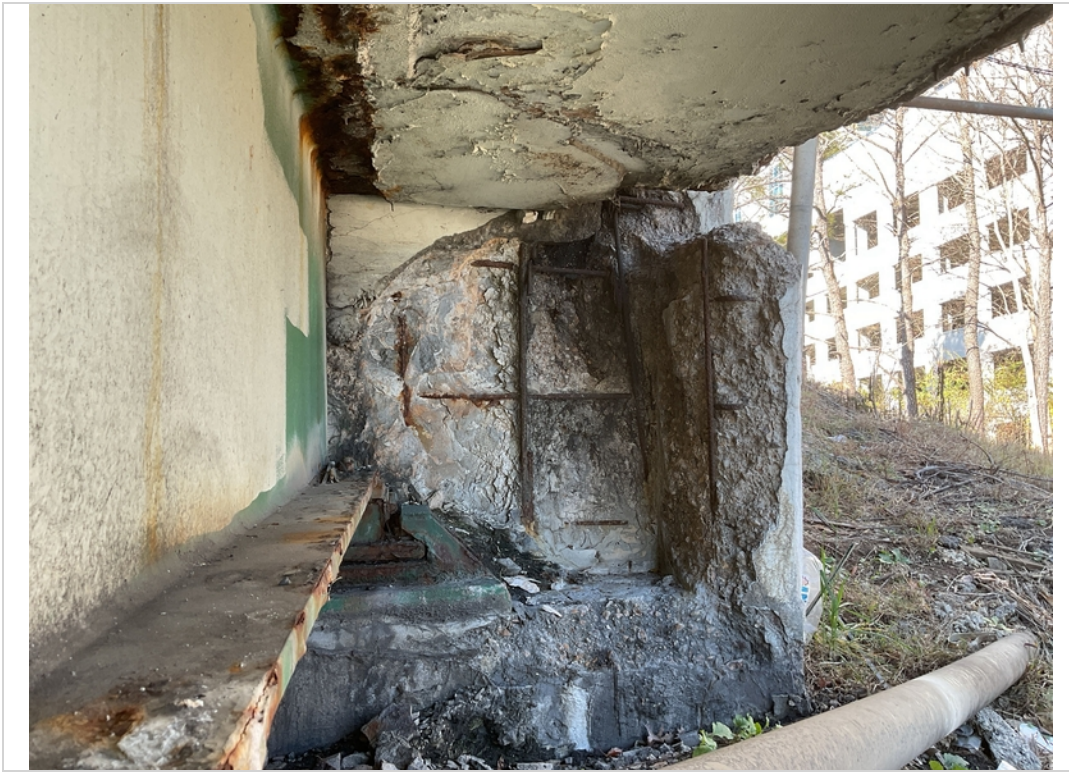
Abut 1 left hvy scale w/exp steel.
