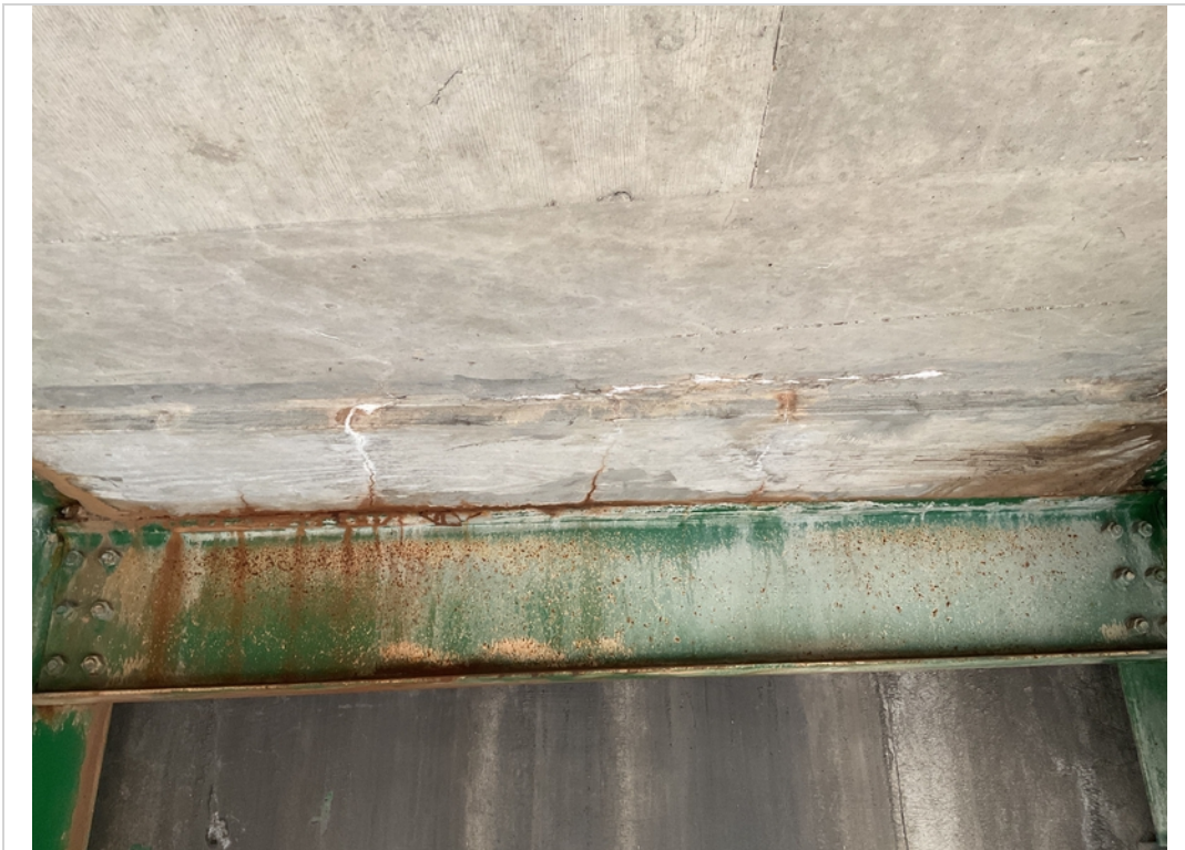
Span 3 bay D failing patch with eff
