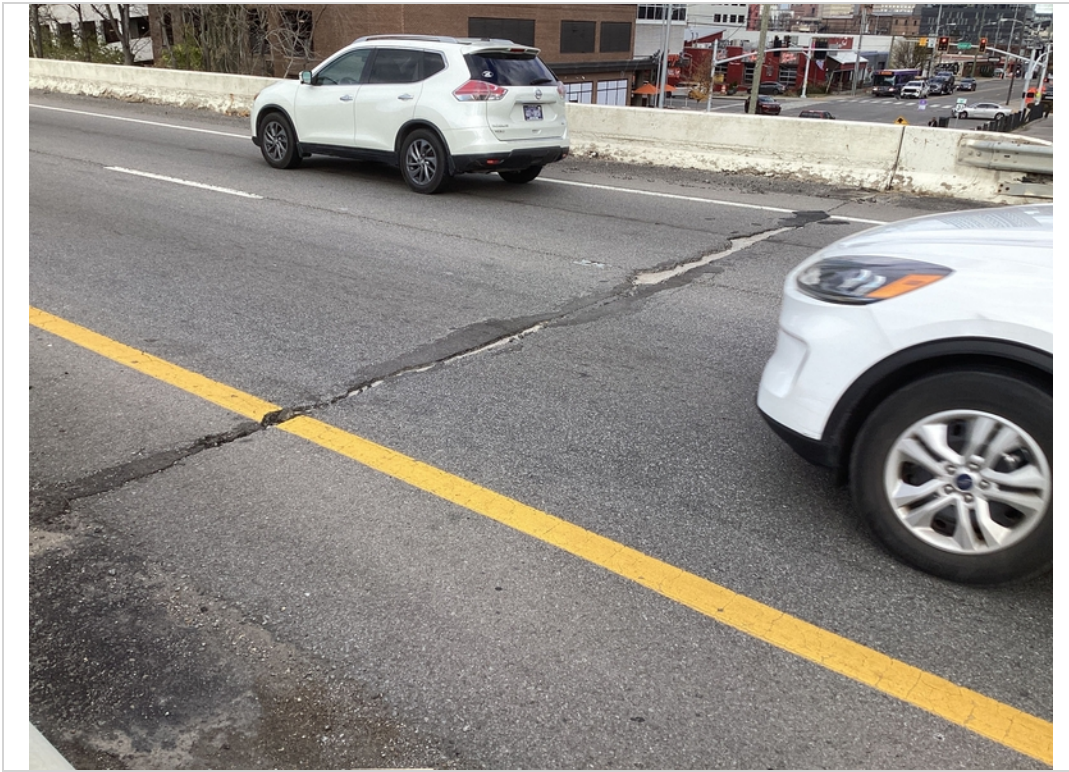
Span 3 joint paved over with light potholes
