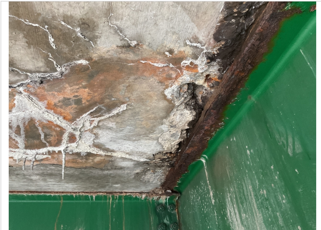
Span 1 bay D failing patch with spalling
